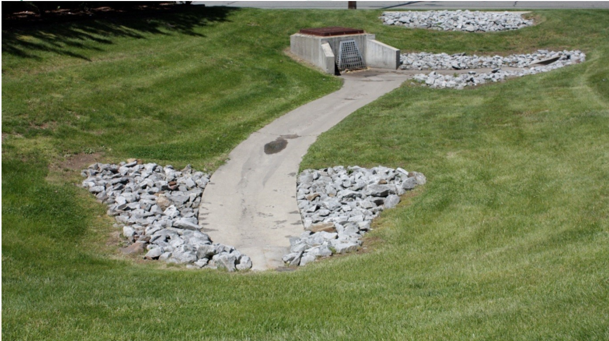
A well-maintained detention basin
